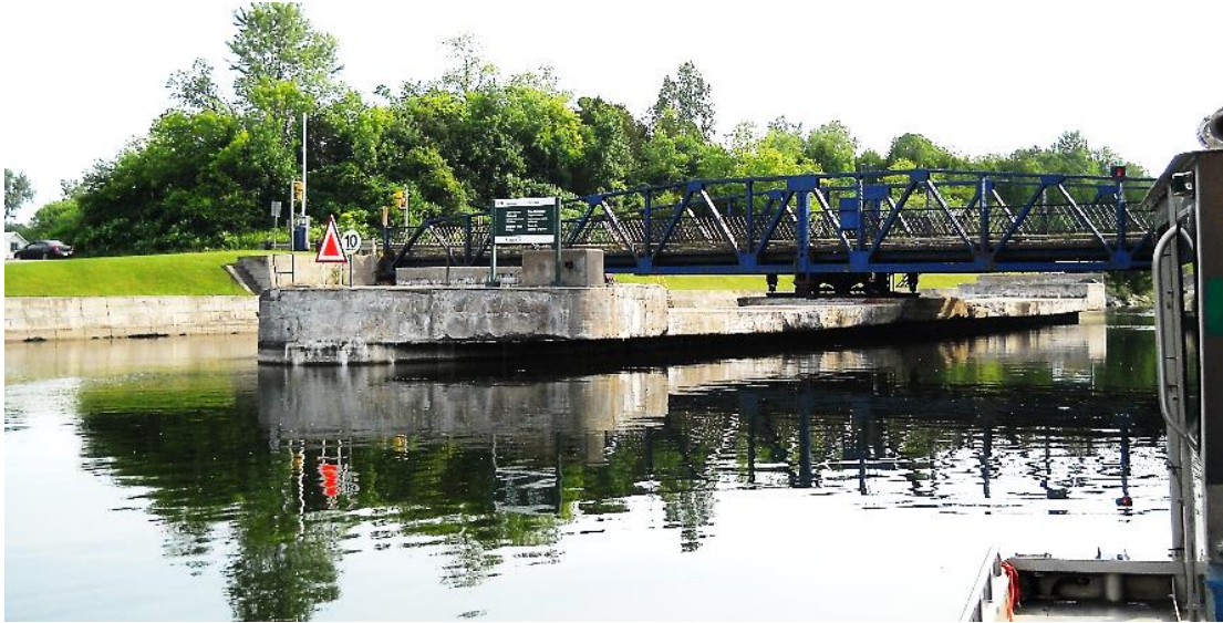
Brighton Road Swing Bridge
